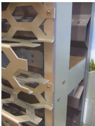
Example: Aluminium profile riveted on bottom plate and perforated panel riveted on aluminium beam
