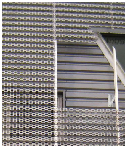
Example: Substructure with screwed aluminium profile angles on bottom plate facade
